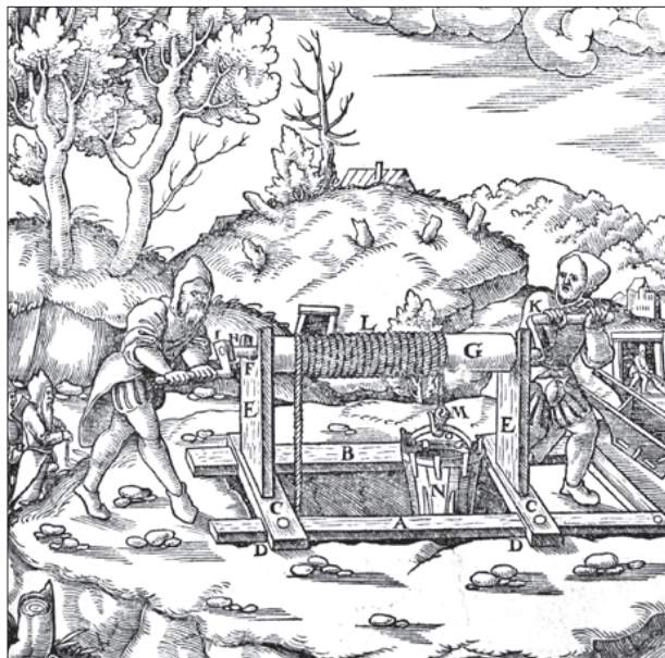
Figure 9. Hand windlass for ore transportation from the mine (haspel-machine) (from Agricola: De re metallica ...).
